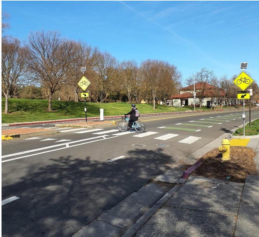
Figure 14: Rapid Rectangular Flashing Beacon (RRFB) on F Street
